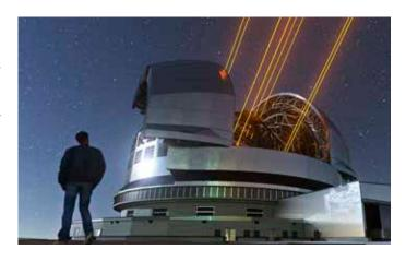
The laser beams (in the photograph) measure the distortion in the atmosphere before light enters the telescope and this is automatically corrected by computers giving the astronomer a clear picture. This telescope, when completed, will be able to collect 100 million times more light than the human eye. Its total mass will be 3000 tonnes.
